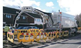
Suction or vacuum excavation (often known as 'vac ex') is a way of safely digging around buried utilities, including gas, electric, water, telecoms and fibre-optics. Being non-aggressive and non-invasive, it's a method of removing the soil, earth or other covering material by means of high-volume air flow.
